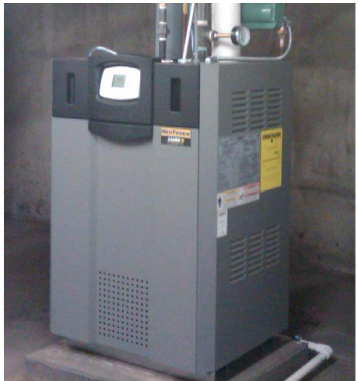
Fig. 3 New condensing boiler
