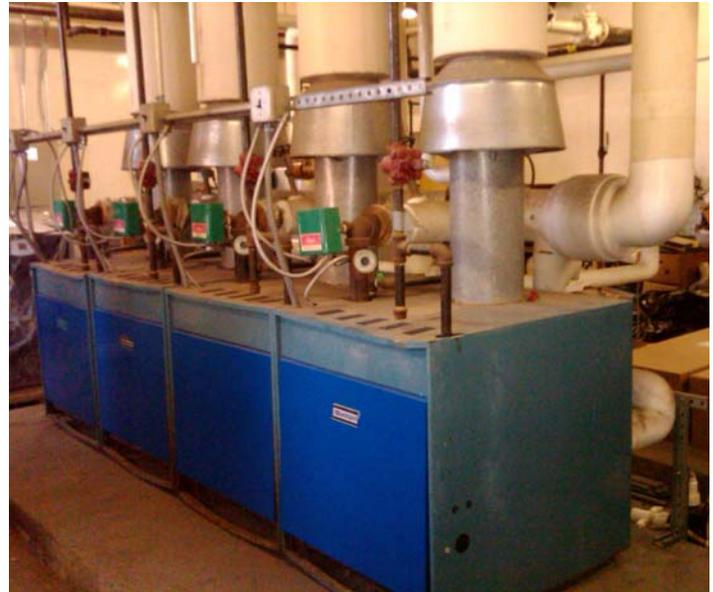
Fig. 2 Cast Iron Sectional Boilers
