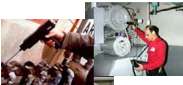
From steam trap faults and valve leakage to compressor problems, ultrasonic detection can be used to find a variety of problems that generate ultrasonic signatures.
