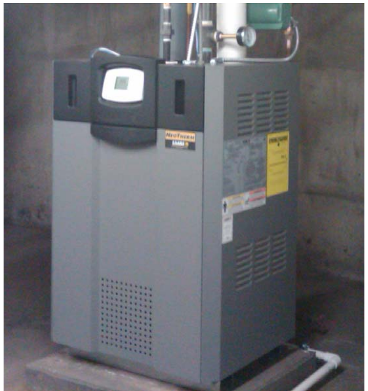
Fig. 3 New condensing boiler
